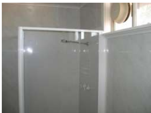
New shower cubicle, tiling, taps and fittings and wall cladding
