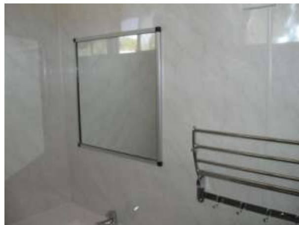
New wall cladding, mirror and towel rack
